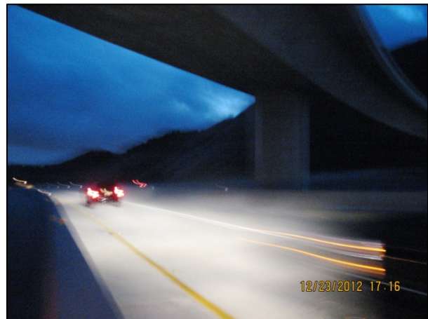
The first car to use the new I-5/SR-14 HOV connector, Dec. 23, 5:16 p.m. Photo taken by Vladimir Gurfinkel, the project's resident engineer.
